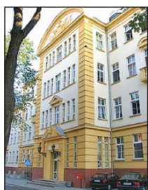
The renovated entrance to Rawicz Hospital
